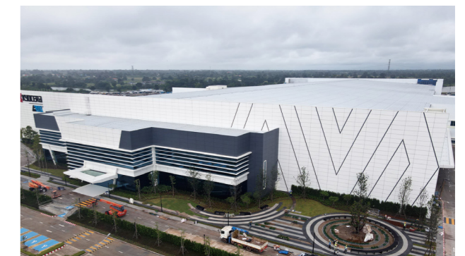
The new KYOCERA AVX Thailand Plant
