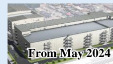
New building at Kagoshima Kokubu Plant
