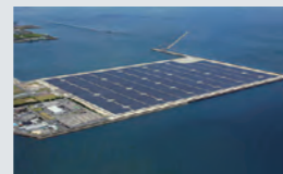
Kagoshima Nanatsujima Mega Solar Power Plant
